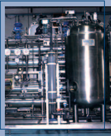
Serbatoio PED per acque pure lt. 3.000 Tank for purified waters lt. 3.000 according PED Drukbehälter PED lt. 3.000 für PW Tank PED lt. 3.000 pour eaux pures
