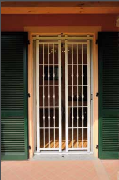
Portafinestra due ante chiusa A closed French window with two shutters
