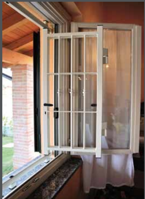
Apertura interna The internal opening
